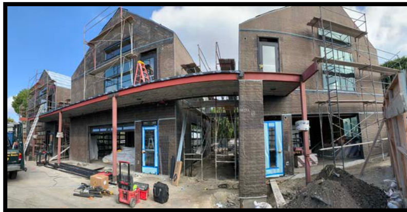
The Center for Innovation under construction
