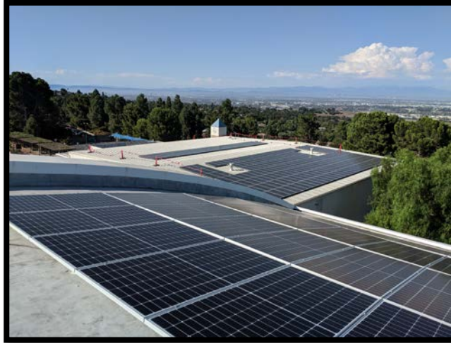
Solar Panels on the performing arts center
