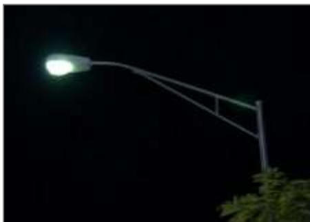
City Of Huntington Beach LED Streetlight Retrofit
